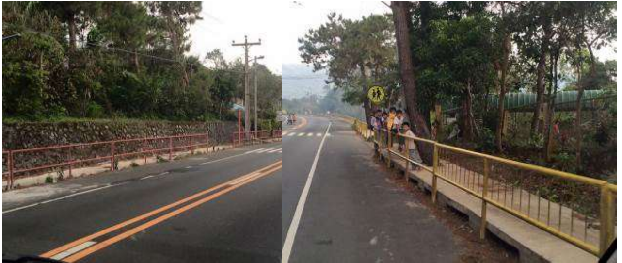
Pedestrian sidewalk installed on newly upgraded shoulder to serve school children
