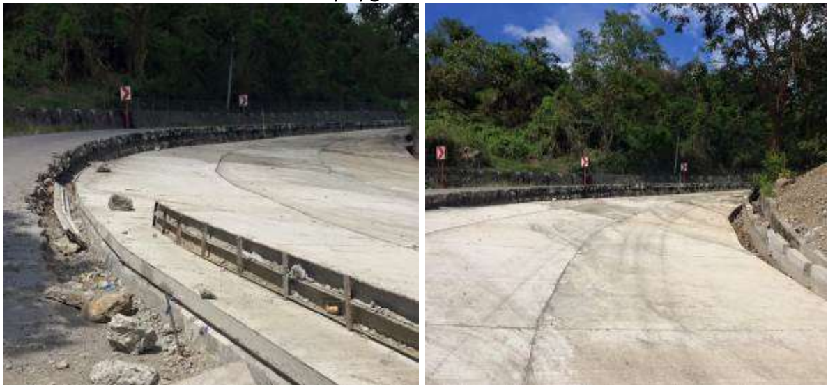
Portion of Case Study Project Still Under Construction
