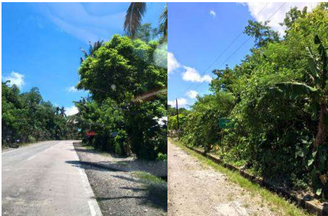
Figure 17. Obstructed Traffic Signs
