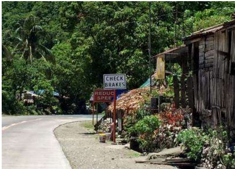
Figure 21. Warning Signs located on the curve
